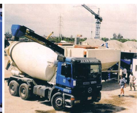
Truck mixer loading belt
